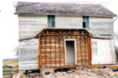
Bailey House - Original location, additions removed - 1997
