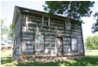
Bailey House - in Lyndon Park - east elevation - 5/24/2010 SJMartin
