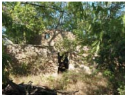
Barn. View to west, looking at east wall. 08/09/2012. KSHS/Hoard, Bob.
