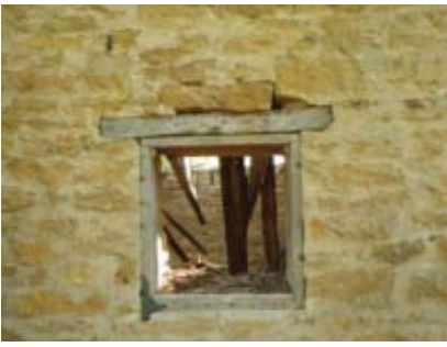
Barn. West wall, window detail. 08/09/2012. KSHS/Hoard, Bob.
