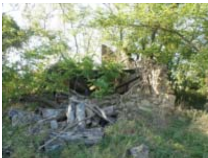
Barn. View to south. 08/09/2012. KSHS/Hoard, Bob.
