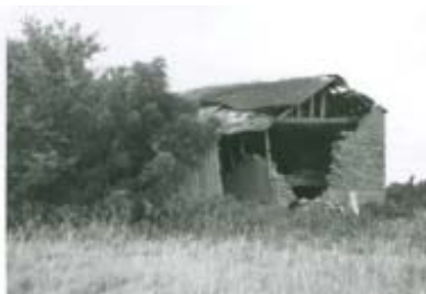
Harris Barn. From NE. 07/27/1971.
