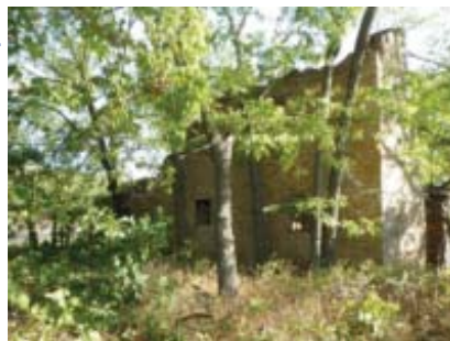
Barn. View to northeast of west wall. 08/09/2012. KSHS/Hoard, Bob.
