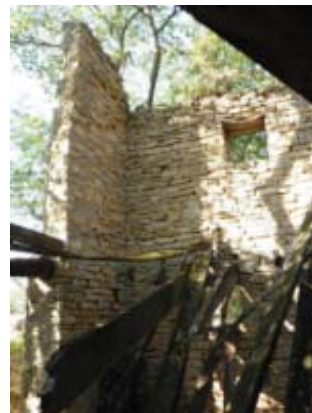
Barn. Interior view to west, showing west wall. 08/09/2012. KSHS/Hoard, Bob.
