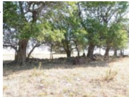
Havana Stage Station Site. Stone fence in trees, looking NE toward station (in background). 08/09/2012. KSHS/Hoard, Bob.
