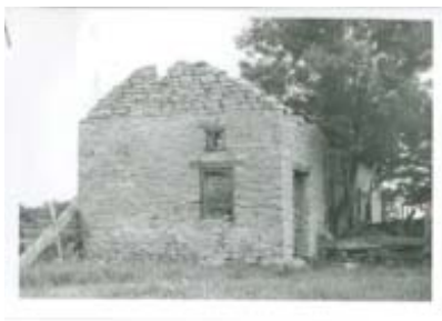
Havana Stage Station. South elevation. 07/27/1971.
