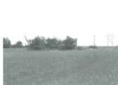
McGee-Harris Station. Station in landscape. 1973.
